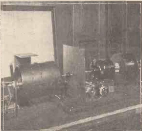
Fig. 9.—Two experimental apertured drums mounted on a common shaft drive.
