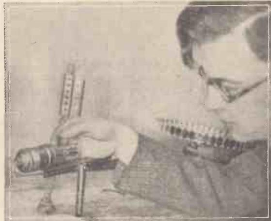
Fig. 14.—A home-made mirror drum shown for use with a crater type neon lamp.
