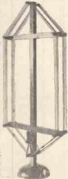
Fig. 9.—A typical commercial frame aerial.
