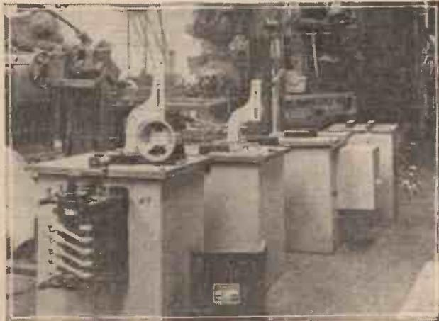
(Above). The corner of a workshop where magnetizing transformers are used with magnet jigs.
