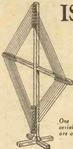
One form of frame aerial in which the wires are arranged in "flat" formation.
