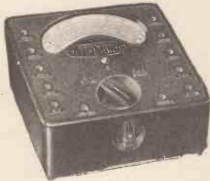
A useful and inexpensive test meter—the Avometer
