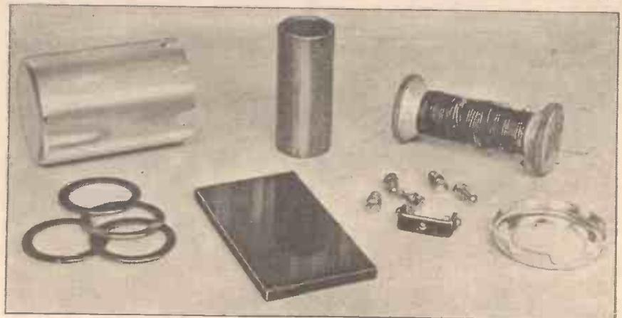
The parts required for the screened coil shown in the heading.
