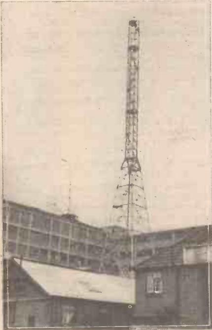
The 200ft. mast to be used for the experimental television service from Hayes.
