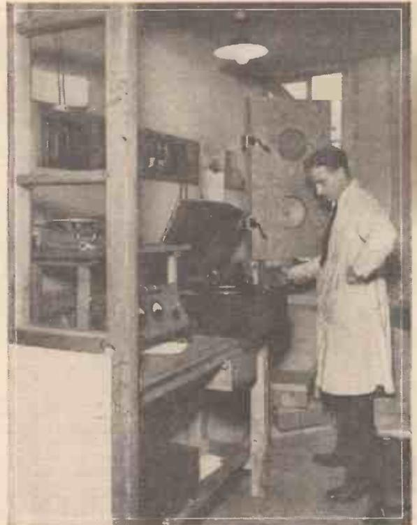
The final listening test for "His Master's Voice" loud-speakers. The loud-speaker which is being tested is compared with one of known performance.
