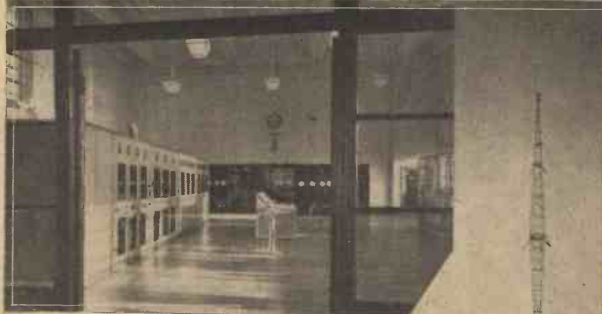
Above may be seen a general view of the transmitter, and on the right a general view of the building and the novel mast aerial.
