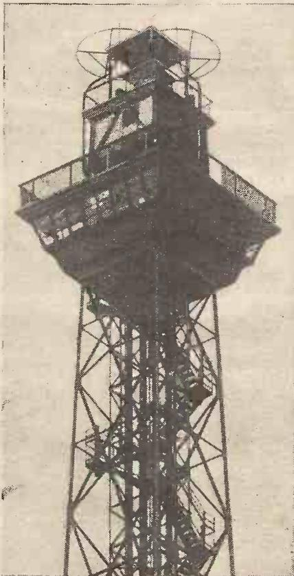
This close-up shows the two dipole aerial arrays on the top of the Berlin Radio Tower. One is used for sound and one for vision, and it will be noticed that the aeri-als are so arranged that the radiation is horizontally polarised.
