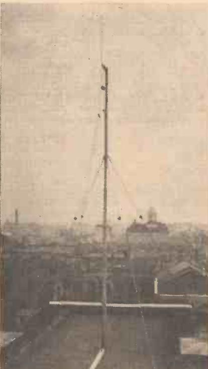
Fig. 1.—A good example of an aerial erection on a roof to secure maximum height.
