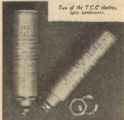
Two of the T.C.C. electrolytic condensers.
