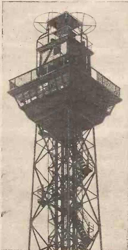
This close-up shows the two dipole aerial arrays on the top of the Berlin Radio Tower. One is used for sound and one for vision, and it will be noticed that the aeriels are so arranged that the radiation is horizontally polarised.
