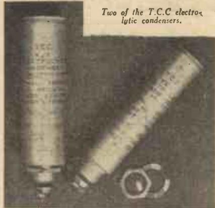
Two of the T.C.C. electrolytic condensers.
