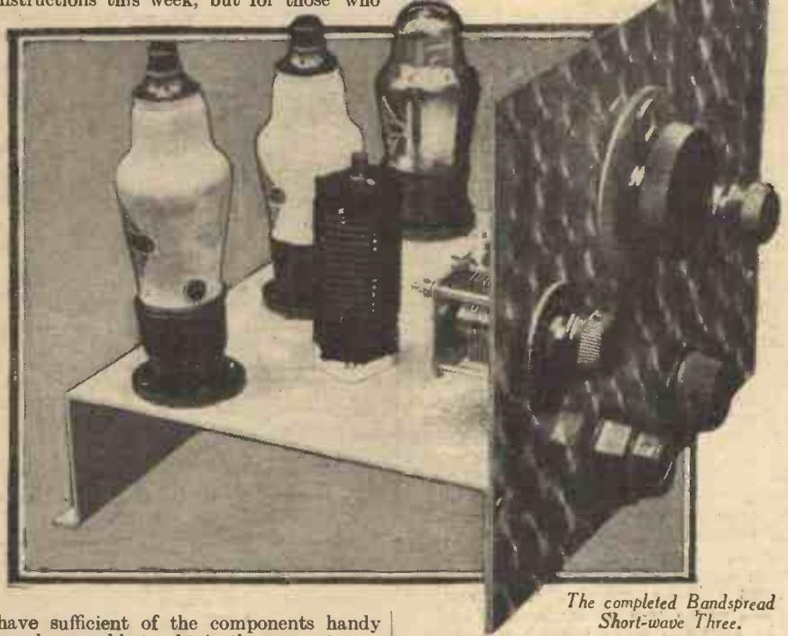
The completed Bandspread Short-wave Three.
