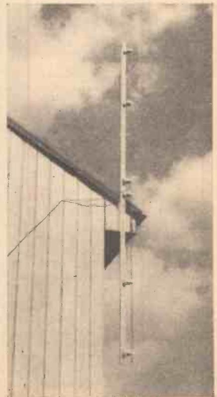
Fig. 2.—A vertical dipole aerial supported by porcelain cleats, and fitted with a flex feeder.
