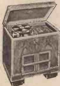
485A-AC. All-wave Superhet Auto-radiogram. 6 valves with AVC. 7-16 (covers Television Sound Transmission), 16.7-53, 46-140, 185-560, 750-2200 metres. **38 GN.**
