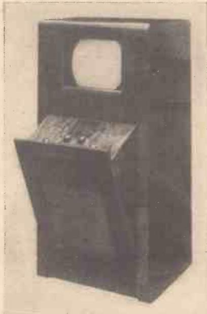
This is the new Baird Model T.11. Note the novel scheme adopted for concealing the radio controls by hinging the lower part of the front of the cabinet.
