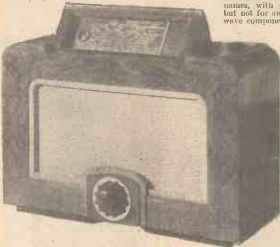
Another interesting feature in dial design seen on the Mullard receiver. Note also how the speaker opening has been centralised and all controls combined in one single knob. The dial may be set at varying angles to facilitate tuning.
