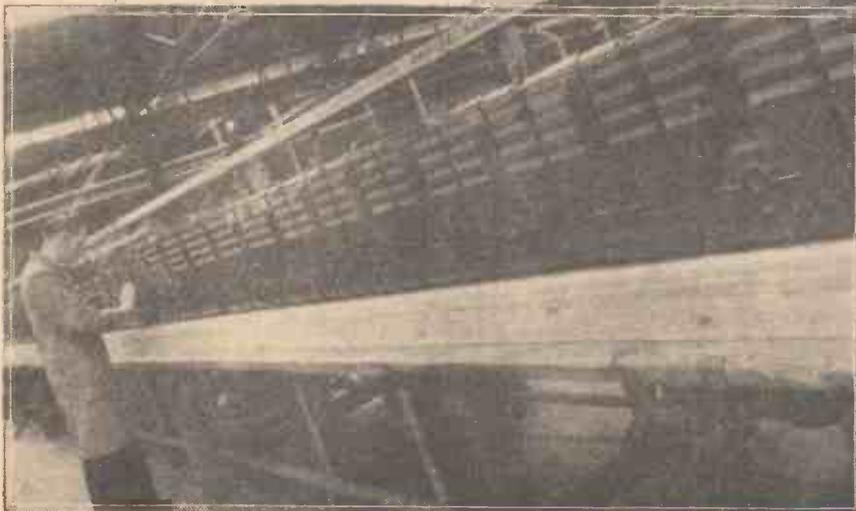
A modern system employed for checking Ekco radio sets—the "Soak" Test. An overhead "live" line supplies A.C. current as the sets move slowly along, towing their mains leads with them. This test under working conditions ensures that all receivers are faultless when they leave the factory.
