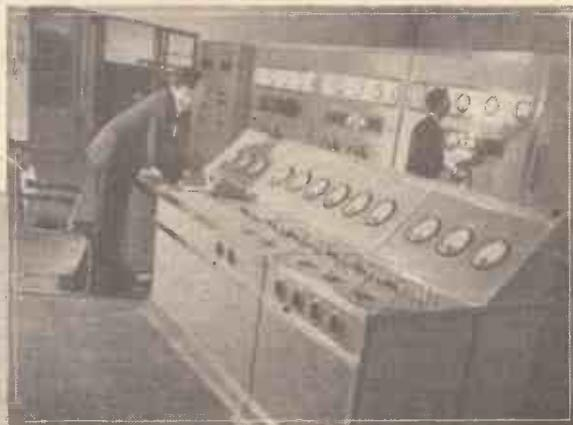
On the left is the vertical mast-aerial, and above is seen the transmitter control desk.
