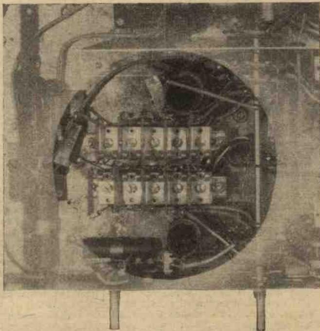
This illustration shows the pre-set condenser assembly in the Invicta receiver shown at the top left-hand corner.
