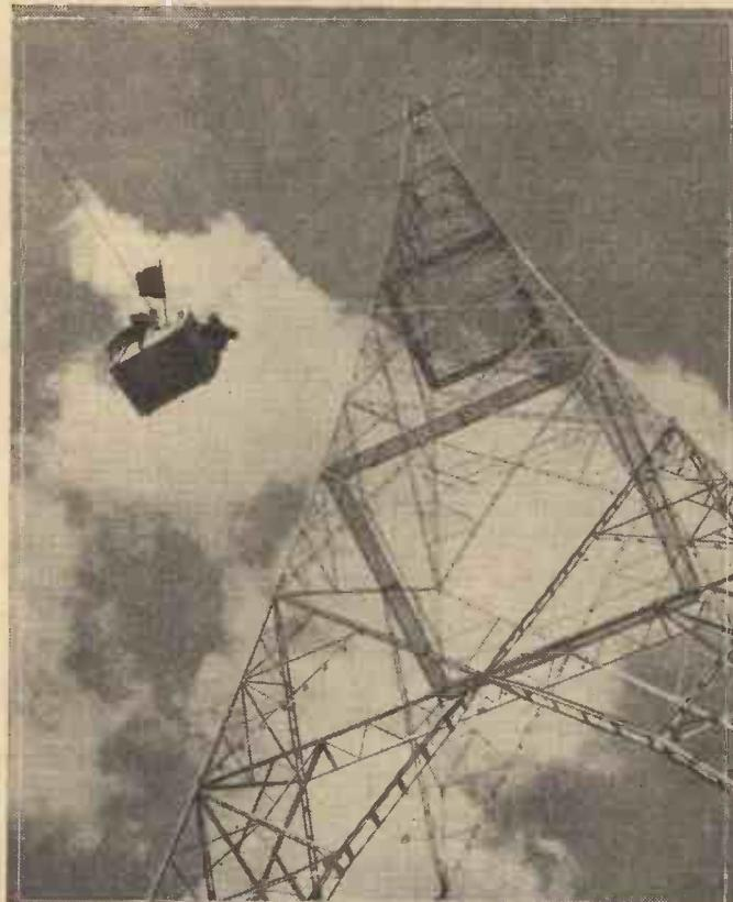
The new aerial tower at Beromünster, constructed by the Swiss engineer, Rudolf Dick, of Lucerne. The illustration shows workmen being hauled to the top of the tower in a wooden cradle.
