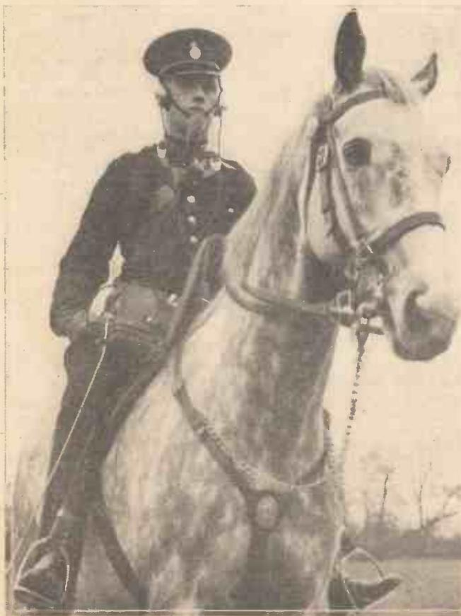
The Grand National crowds this year were controlled by mounted police equipped with radio. Messages were received from a central headquarters on an aerial, which is seen in the illustration, depending from the receiver, which is strapped to the saddle.
