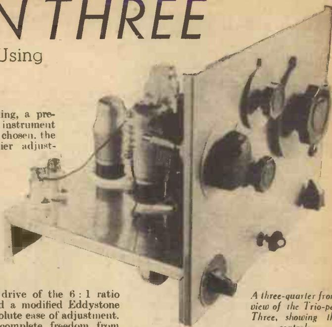
A three-quarter front view of the Trio-pen Three, showing the controls.
