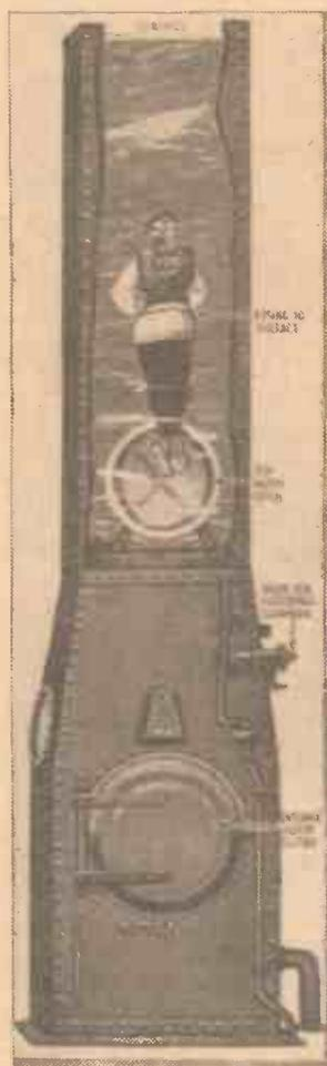
A training tank with latest type of escape lock, as built in new submarines in the British Navy.
