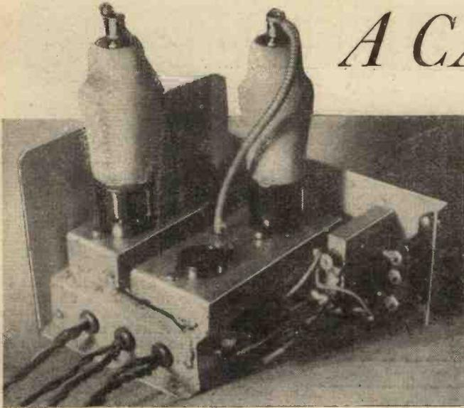
Fig. 8.—General view of the experimental time-base chassis.
