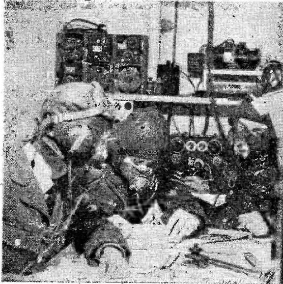
An air crew of the R.A.F. using a cubicle representing an aircraft in which they carry out operational flights on the ground.
