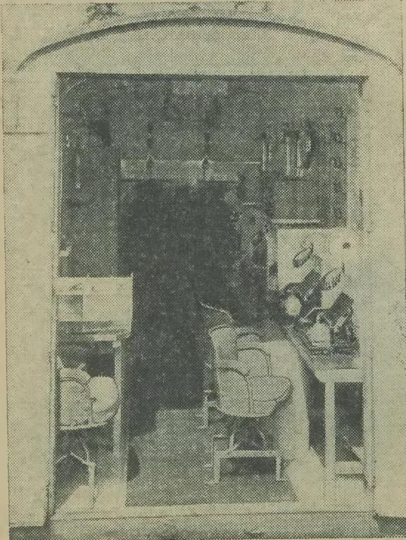
View of receiving vehicle. Reading right to left are two perforating positions, one undulator with receiver and bridge above, one Wheatstone transmitter, then second undulator with second receiver above and two tape reading positions. Desk on front left is the superintendent's desk.
