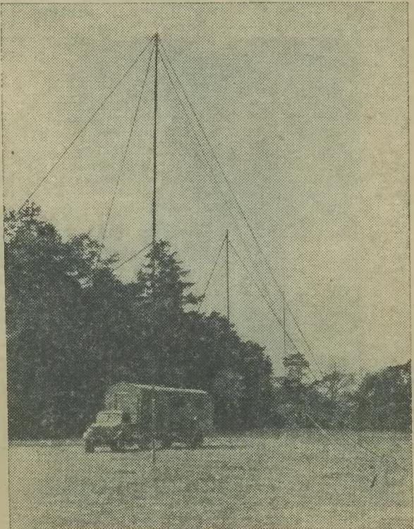
The receiving vehicle and 70ft. aerial masts. The transmitting van is usually located some distance away and operated from the receiving vehicle by means of a suitable cable line.
