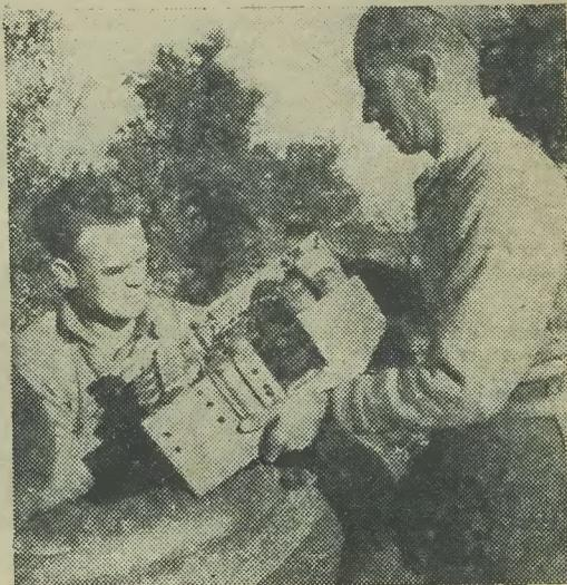
When a damaged wireless set arrives at the R.E.M.E. wireless depot attached to the 8th Army it is repaired and tested for service again. The illustration shows a repaired set being inspected prior to its reinstallation in a Sherman tank.
