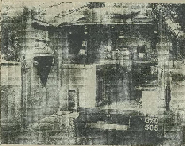
A B.B.C. recording truck, as used by B.B.C. war correspondents. Interior view, showing single channel recording apparatus. Short-wave receiver can be seen on the right and three channel mixer and loudspeaker above.
