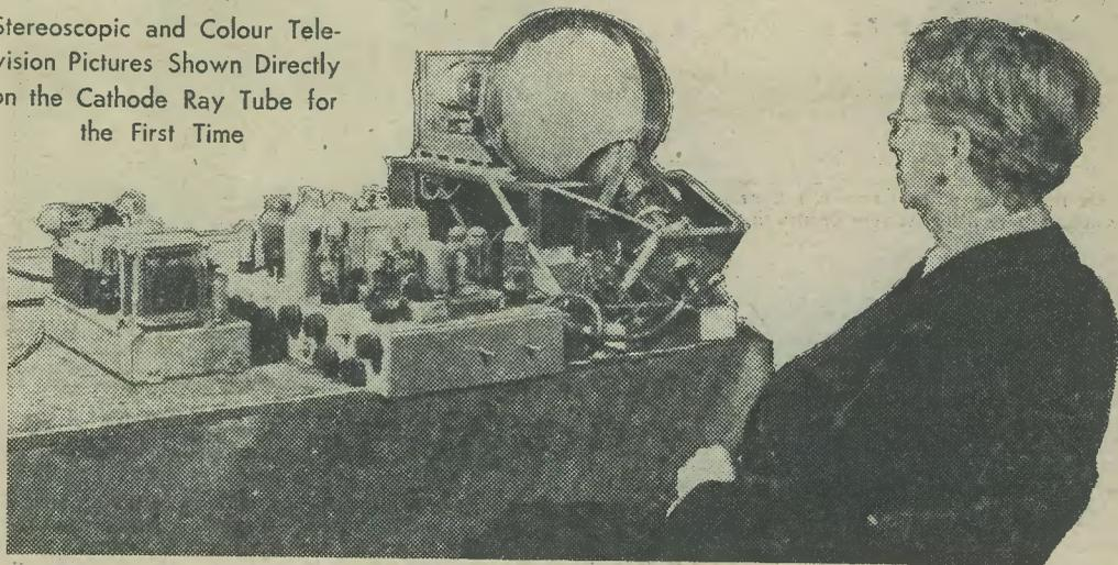
Fig. 1.—Photograph showing Mr. J. L. Baird looking in on the "Telechrome," his latest invention. The "Telechrome" is a cathode ray tube which shows television in colour and also in stereoscopic depth.
