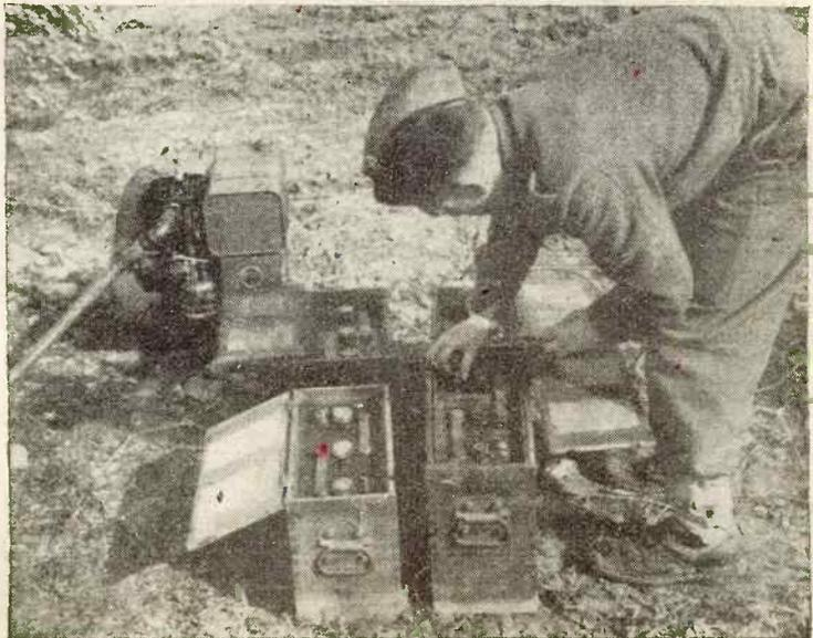
*With the Royal Corps of Signals on the 8th Army front in Italy. An electrician connecting up batteries to a small petrol-driven generator which charges the batteries for wireless sets at H.Q.*
