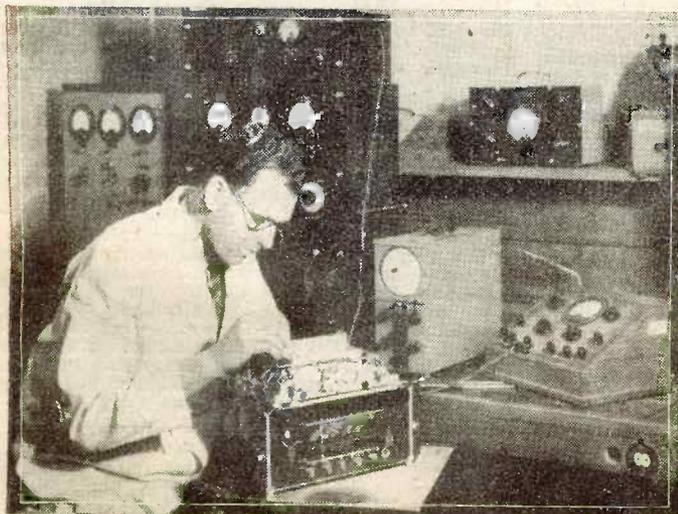
*Final testing of factory-produced receivers and transmitters is a very important and interesting job for well-qualified engineers. A considerable amount of highly-developed test equipment is required.*
