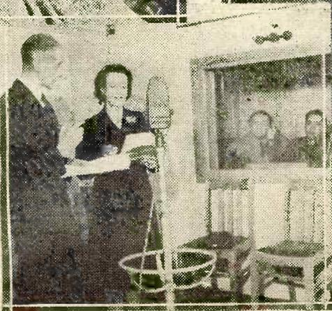
*Above: Gramophone Unit Operation. A student from the School Broadcasting Department learns how to mark up a disc. Using a yellow chalk pencil, sharpened to a fine chisel edge, she is marking a groove in which a certain sound effect is recorded. By means of headphones she can hear the effect being played as she marks its exact position on the disc.*
