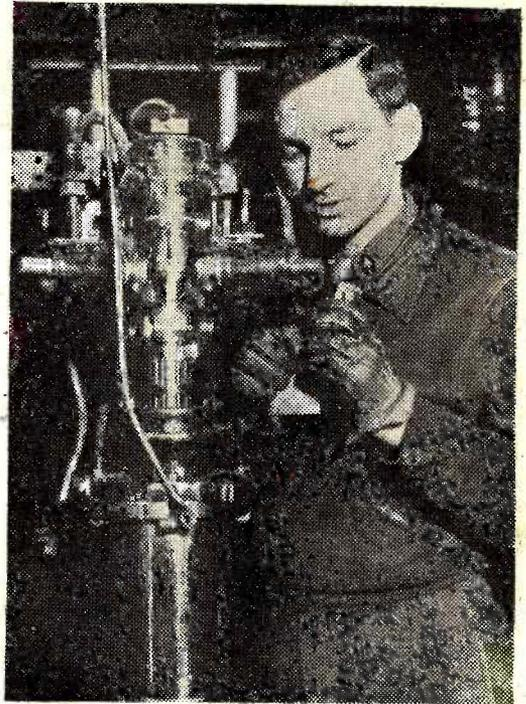
*After going off the air when the Germans advanced into Luxembourg, this station was dismantled, but started operating again at the end of last December. The illustration shows a radio engineer making a final connection to one of the high-power valves.*
