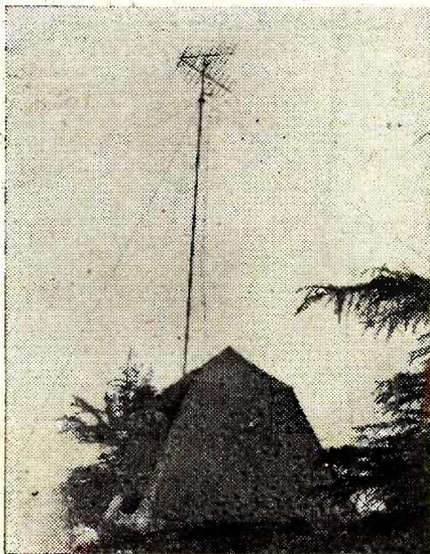
Fig. 19.—A television relay station in a tent, used by the Don Lee station in California to carry programmes back to the transmitter for rebroadcast to the public.
