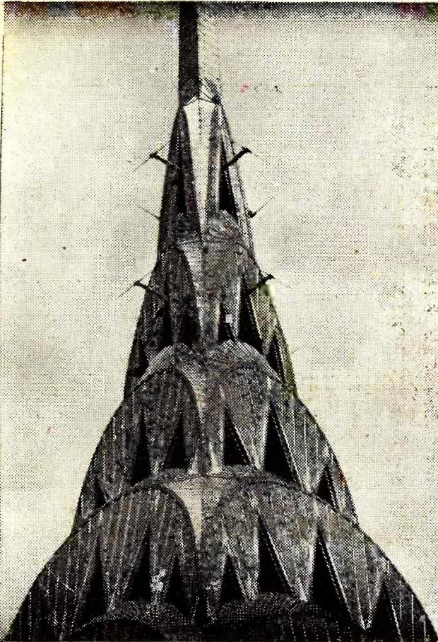
Fig. 21.—The transmitting radiators of the C.B.S. transmitter in New York, on top of the Chrysler Building (elevation 1,046 ft.).
