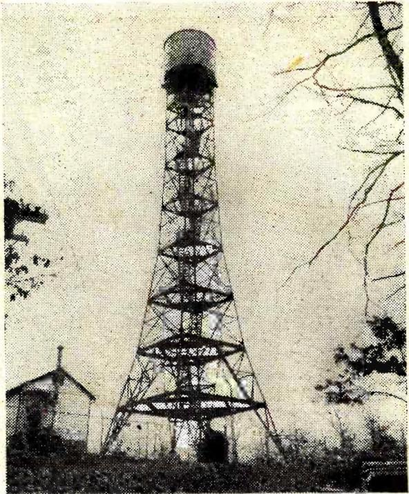
Fig. 20.—An elaborate television repeater station, constructed by R. C. A. Communications to relay programmes from Long Island to New York. The picture signal is sent by frequency modulation in this equipment.
