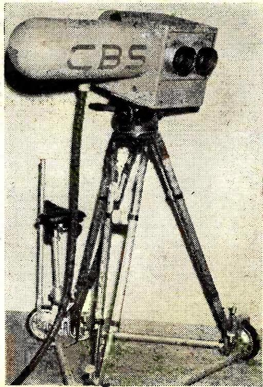
Fig. 23.—Orthicon colour-television camera developed by P. C. Goldmark, of C.N.S. The housing contains a rotating optical filter system to produce successive images in the three primary colours.
