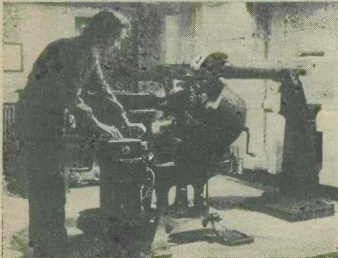
*In this equipment the standard cine film is projected direct into the television camera. The film is used as a fill-in in broadcast plays, etc. Trainee Mrs. Dorothy Jones is operating the apparatus.*
