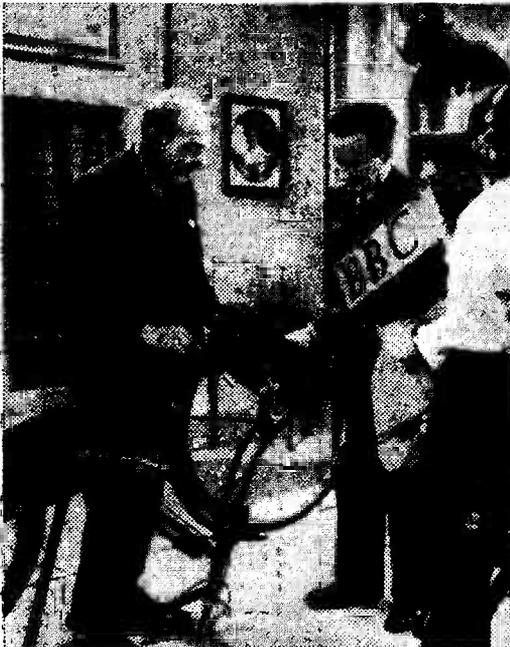
*P.A.Y.P.! Pump as you pedal! Mr. F. J. Camm's new invention, an automatic tyre pump, being televised for "Picture Page". It incorporates a check valve which blows off when correct pressure has been reached, and will keep the tyre inflated even with a slow puncture.*
