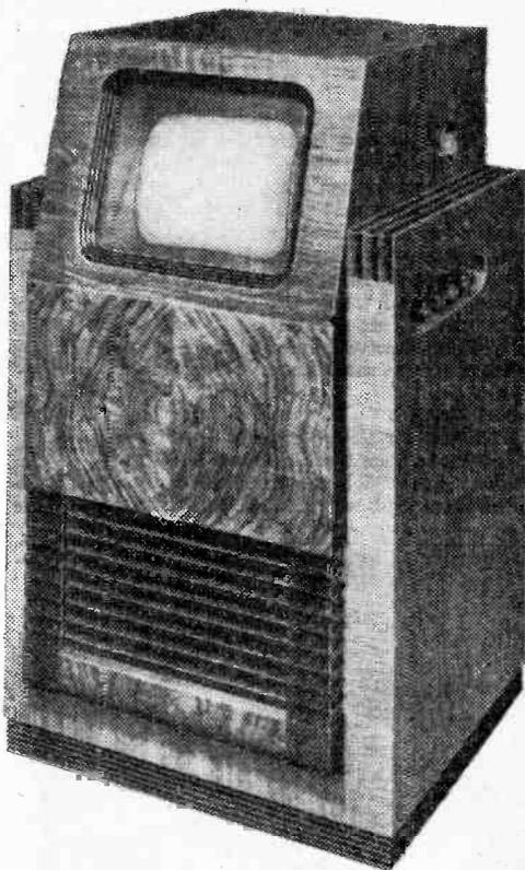
*This television receiver by R.G.D. has a Thyatron time-base and employs magnetic scanning. It gives a 10in. by 8in. picture.*
