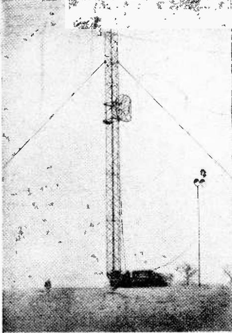
*The temporary masts on which the paraboloid aerial can be raised or lowered. The smaller portable mast is used for contact between the two mobile laboratories.*
