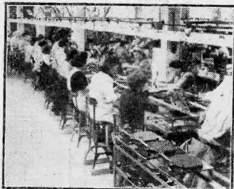
A section of the automatic record-changer production line in the Plessey Co.'s works at Ilford.
