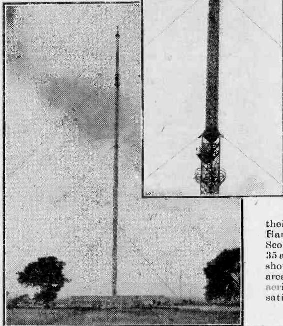
The transmitter building at Sutton Coldfield and its 750ft. mast. The wide-band aerial at the top of the mast is shown inset.
