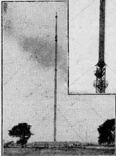
The transmitter building at Sutton Coldfield and its 750ft. mast. The wide-band aerial at the top of the mast is shown inset.
