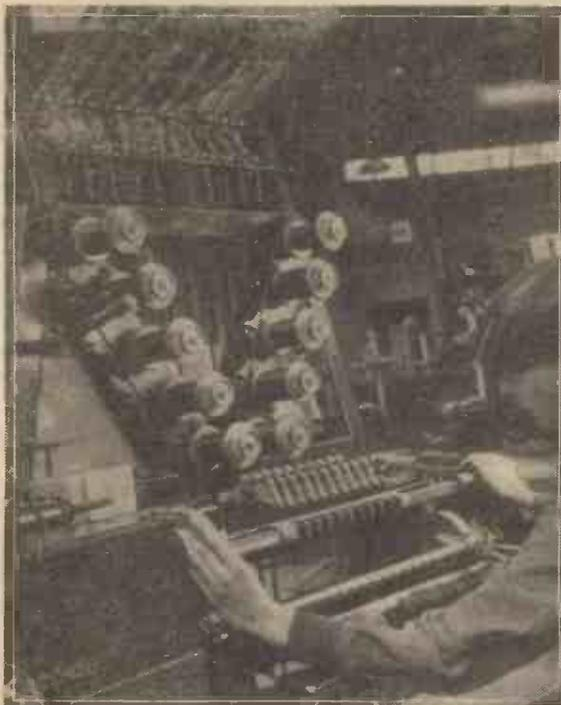
The set maker overcomes a difficulty. Here is an ingenious machine which winds 10 coils at a time, under the control of a single operator.
