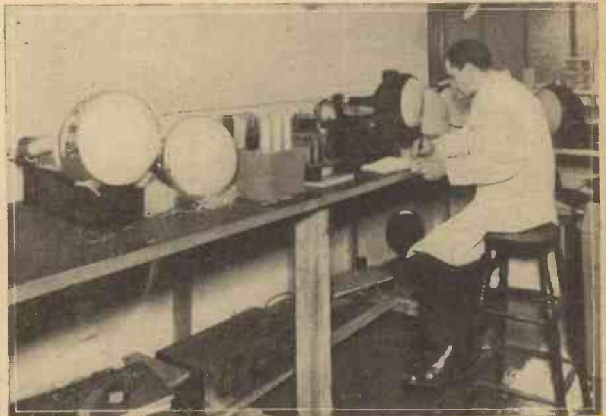
Cathode-ray tubes undergoing one stage in acceptance tests, particularly in regard to the degree of contrast range exhibited.
