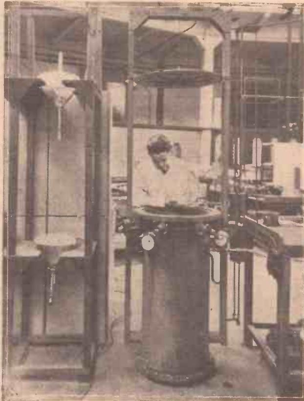
An important part of cathode-ray tube manufacture is the final pressure testing, and the illustration shows a tube about to undergo this process.
