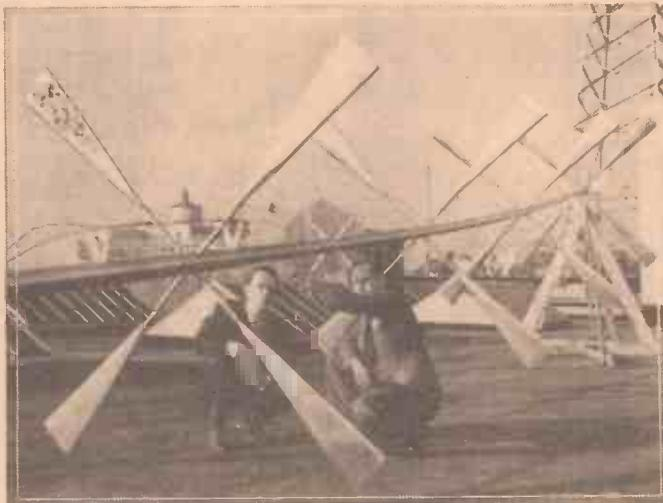
An unusual type of television aerial which was experimented with in America. It was claimed that better definition could be obtained by means of the paddle-like elements.
