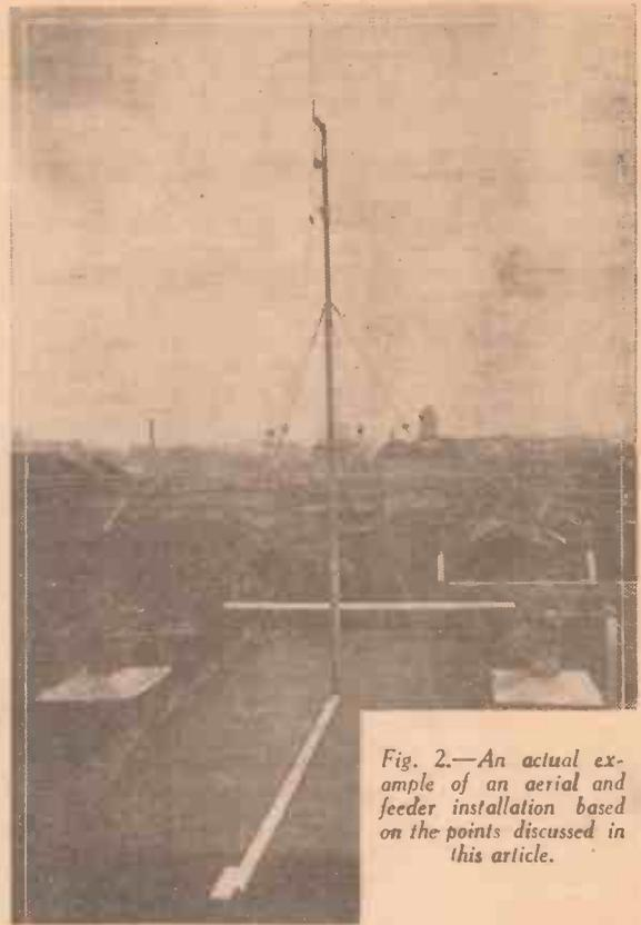
Fig. 2.—An actual example of an aerial and feeder installation based on the points discussed in this article.
