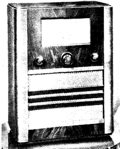
Model 35.—4-valve All-wave Cossor battery superhet.
