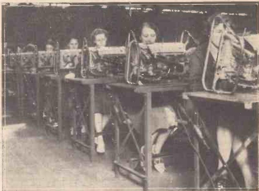
A view of the production desks in a modern radio factory, showing motor-controlled receivers nearly ready to leave their "cradles" for assembly in their cabinets.
