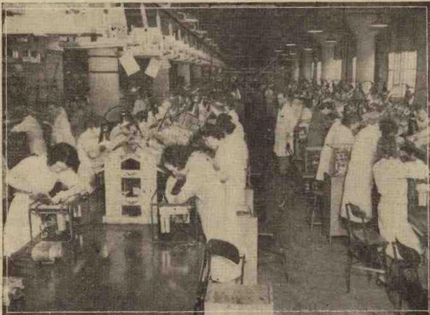
One of the shops where the machines start with small parts and finish up complete wireless sets for export. Each section is responsible for a particular section. Note the overhead trolley with completed wireless sets en route to the packing department.
