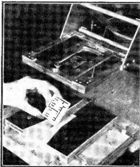
A "wired" chassis. The main part of the American miniature receiver in which wiring, resistors, etc., are all chemically printed with oxide silver paint on ceramic.
