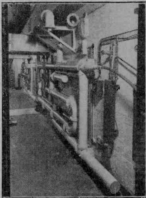
The vestigial sideband filter, constructed of lengths of concentric feeder, which is connected between the output of the vision transmitter and the feeder to the aerial at Sutton Coldfield. The filter is of the constant-resistance type and comprises a high-pass and low-pass section.
