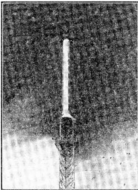
*The cylindrical upper portion of the 360ft. mast at Wrotham. This section is 110ft. long and 6½ft. in diameter, and forms the V.H.F. aerial proper.*
