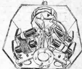
Coil Pack in carton with instructions. Pre-aligned. Post Free **19/6**. Ranges covered: 15 to 50 metres and 200 to 500 metres.
