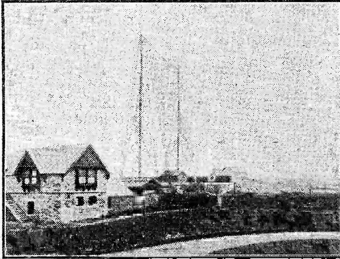
170ft. masts with 60 wire fan-shaped aerial at Poldhu, used for Marconi's first Trans-Atlantic experiment in 1901. A power of 12 kW. was used.
