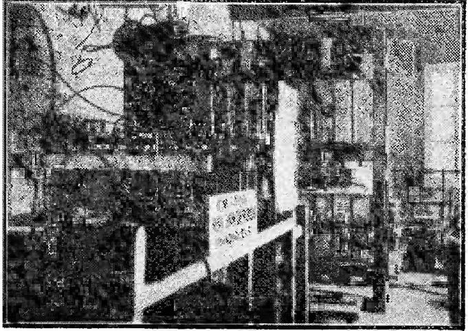
*Some of the early apparatus at the Poldhu Wireless Station. On the extreme left are the transformers. The banks of condensers are carried in metal containers in the wooden rack. On the extreme right is the spark gap consisting of two steel spheres mounted on insulating rods. Used in sending first Trans-Atlantic signals, 12th December, 1901.*
