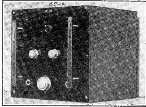
The completed amplifier for rack mounting.
