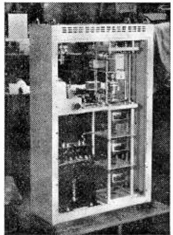
One of the voltage regulators made by Foster Transformers for the BBC.
