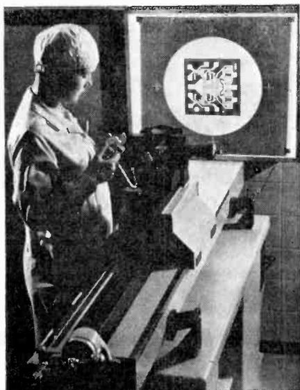
◀ Here, under very clean conditions, a high-precision camera is being used to photographically reduce a large scale drawing of an integrated circuit mask.
