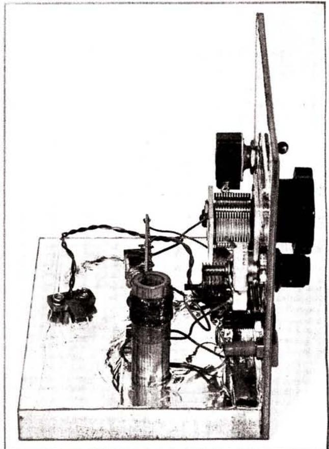
the variable capacitors' fixed vanes and antenna and earth sockets. The switch, output socket and battery connector leads may now be wired to the Veroboard. The wiring is checked, battery and headphones connected and the power switched on. If a loud hum emanates from the headphones when a finger is placed on C3 the circuit is probably functioning correctly.
