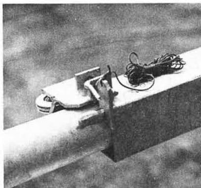
**Installing the UM1. On the left: plumbing the ground-post (top); the bolt locking the mast sections for tilting (centre); toggle catch with nylon operating cord (bottom). And above: UHD-2, KR-400 and antenna installed (top); job completed—mast upright! (bottom)**
