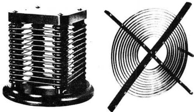
Fig. 1: Early forms of transmitting tuning coils
