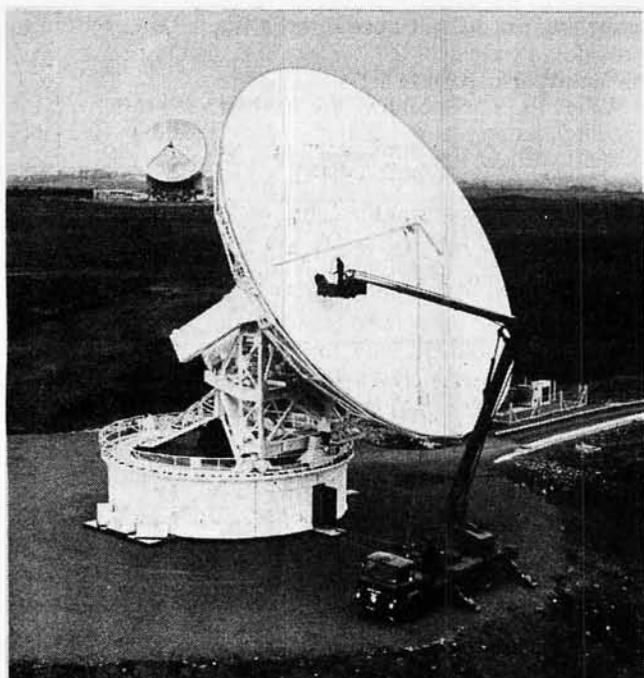
**Fig. 2.3: British Telecom's Goonhilly 4 antenna being prepared for 11/14GHz operation**
