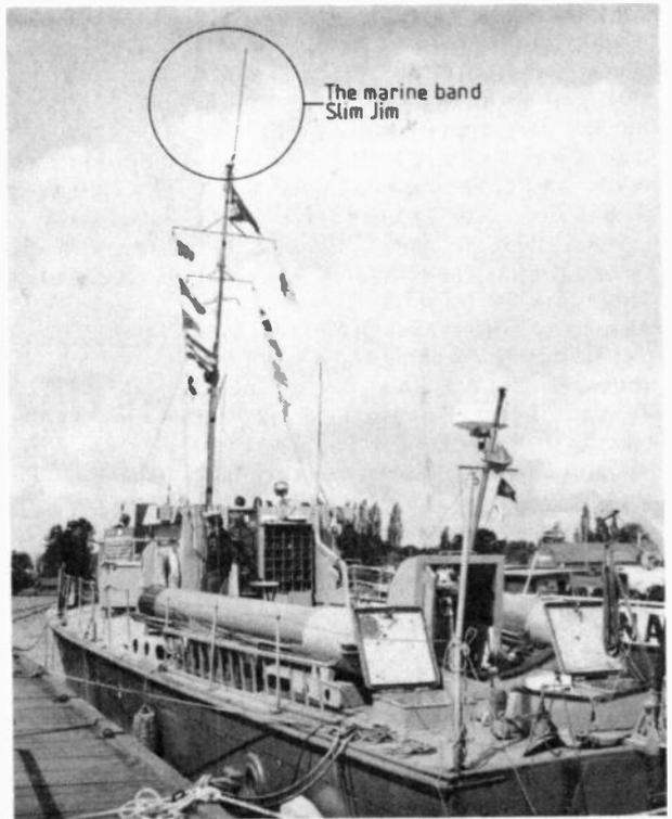
Fig. 1.4: Marine band "Slim Jim" mounted at the mast top of a renovated ex-WWII Motor Torpedo Boat
