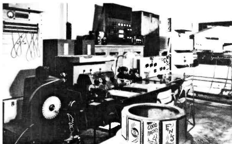
**Fig. 4: The BBC television control room at 16 Portland Place in London in 1935. Caption machine in foreground, with disc scanner on the left, with twin monitor receivers above. The mirror-drum scanner (the camera) is pointing into the studio.**
