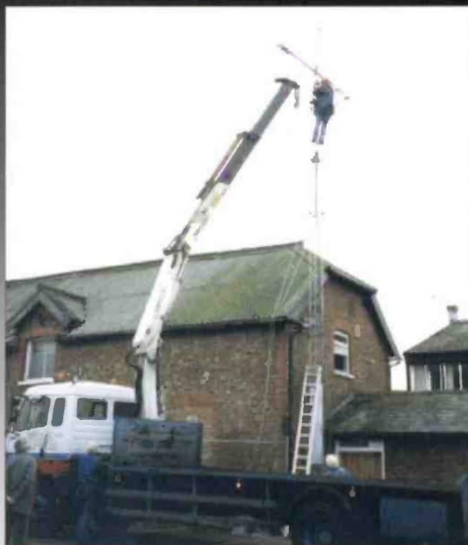
Warrington ARC were busy this summer when some misleading information from their planning authority meant that after having erected their Force 12 array on a fixed mast, they were ordered to then mount it on a retractable mast so that it could be 'parked' at roof level.
