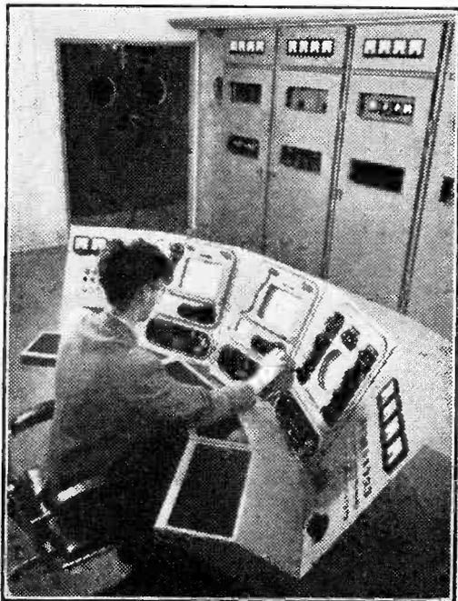
The control desk for the medium-power stand-by transmitters, parts of which may be seen in the background. These have a power of 5 kW. (vision) and 2 kW. (sound).
