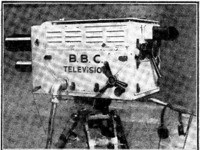
The C.P.S. Emitron camera, with electronic viewfinder. The lens turret is controlled from the rear.
