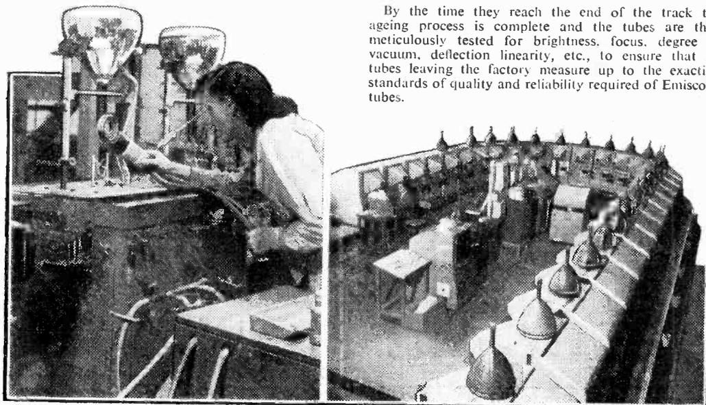
On the left is shown Modulator Outgassing process, whilst on the right may be seen the railway carrying the tubes for the ageing and testing process.
